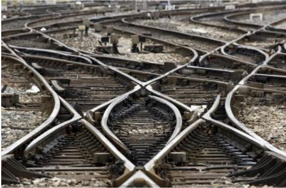
Figure 15: row of track equipment around the Brétigny train station
